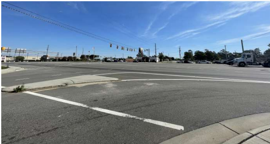
The ‘Point’ in Spring Lake where NC 87 and NC 210 split. Pedestrians have to cross 14 lanes of traffic to get across Town.
