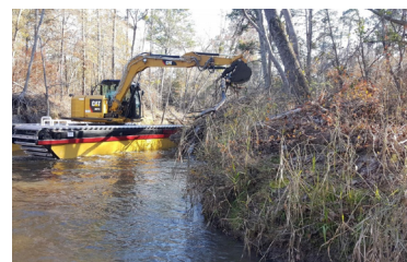
Amphibious equipment removing vegetative debris from stream channel
