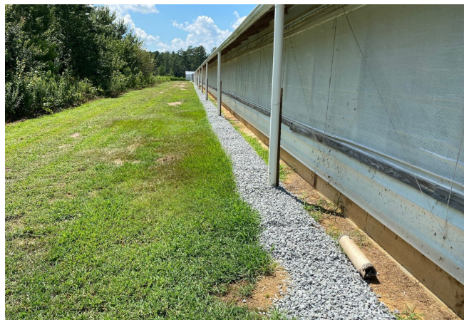
Roof Runoff Structures are installed to prevent erosion around animal agriculture operations.
