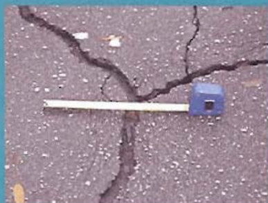
Severe Pavement Crack
