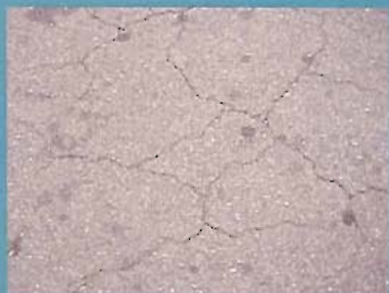
Alligator Cracking
